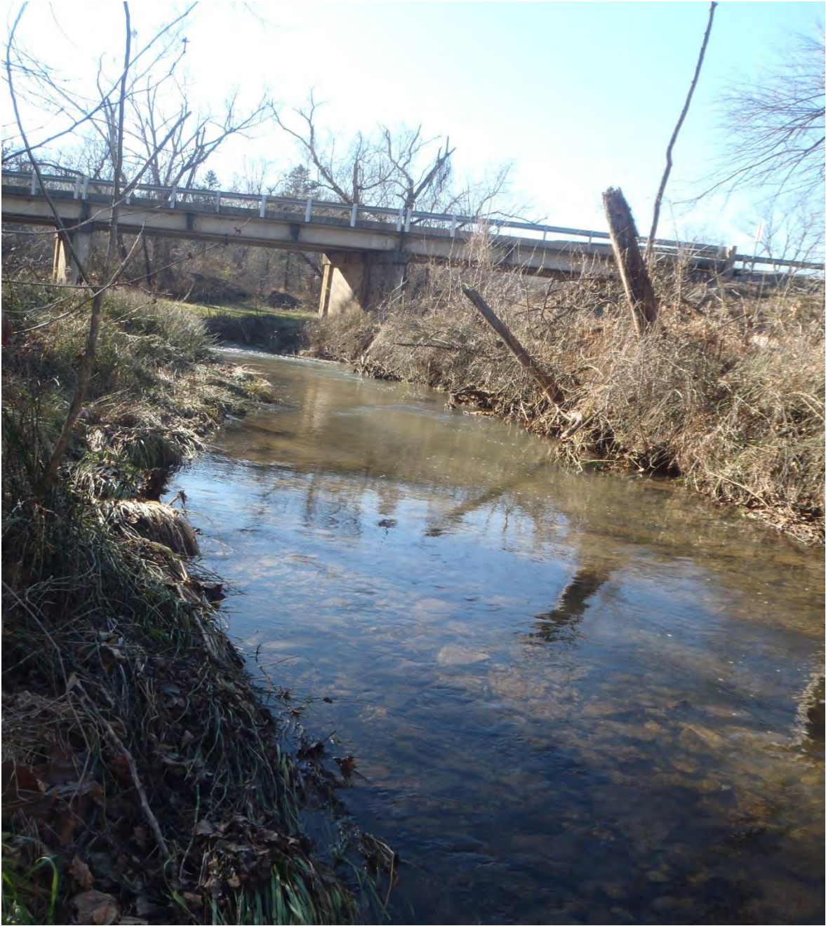
Looking upstream at existing Mill Creek Bridge
